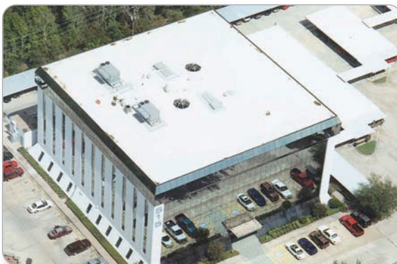
Complete roofing system
